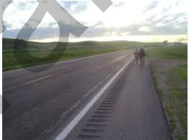
Paved shoulder with rumble strip. Source: Small Town and Rural Multimodal Networks , U.S. DOT FHWA..
