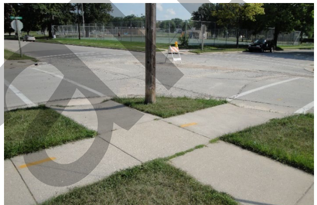
Perpendicular curb ramps aligned with crosswalks.
