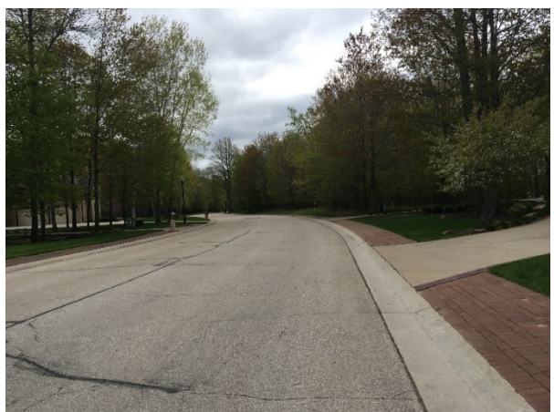
Example of an existing neighborhood street in Thornberry Creek Estates.
