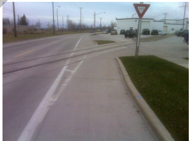
Railroad crossing requires enough room for bicyclist to approach the tracks at 60-90 degrees.
