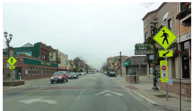
Speed table/elevated crosswalk in a commercial area. Source: Urban Street Design Guide, National Association of City Transportation Officials.
