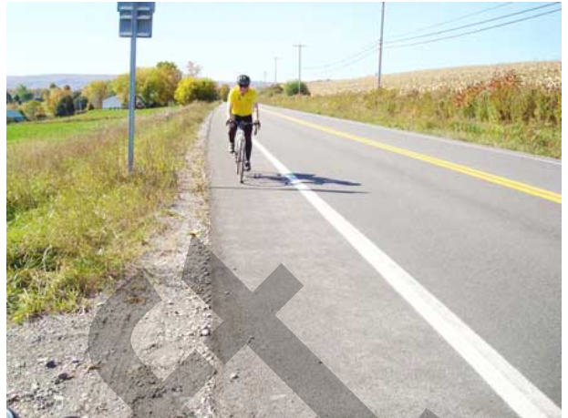
Paved shoulder. Source: Cornell Local Roads Program.
