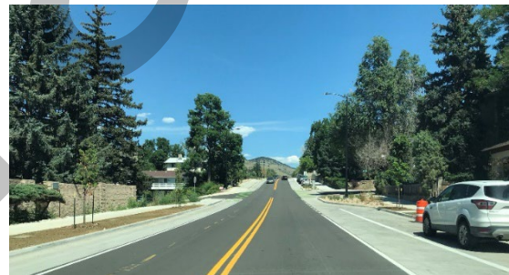
Bike lanes and parking lane contrast with the roadway, further delineating the spaces. Golden, CO.
