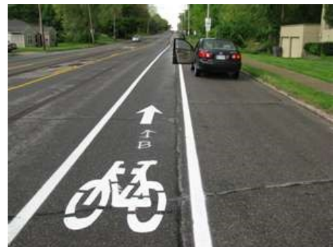
Parking lane is designed to include the car door, limiting the chance of a cyclist hitting an open door.
