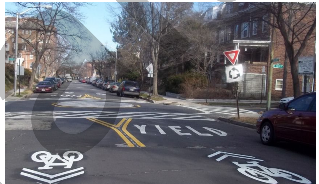
Mini roundabout with mountable apron and island that larger vehicles can drive over to negotiate turn. Source: Urban Street Design Guide, National Association of City Transportation Officials.
