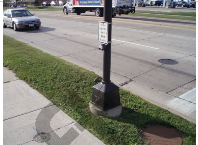
Example of a pedestrian signal activation button that is reachable from the sidewalk.
