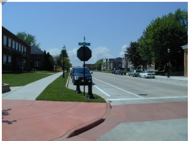
Curb extension at the Grant Street/Fourth Street Intersection in De Pere.
