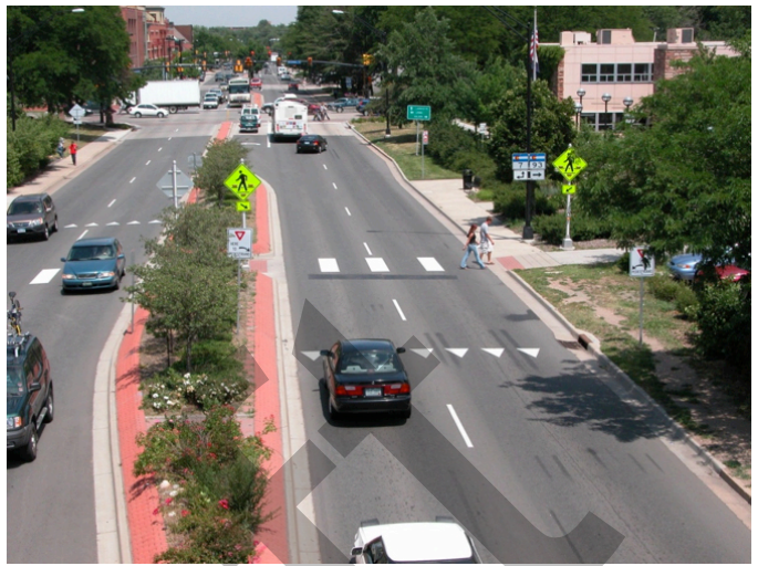
Advance yield markings at midblock crosswalk with a refuge island. Source: pedbikeimages.org – Toole Design Group.
