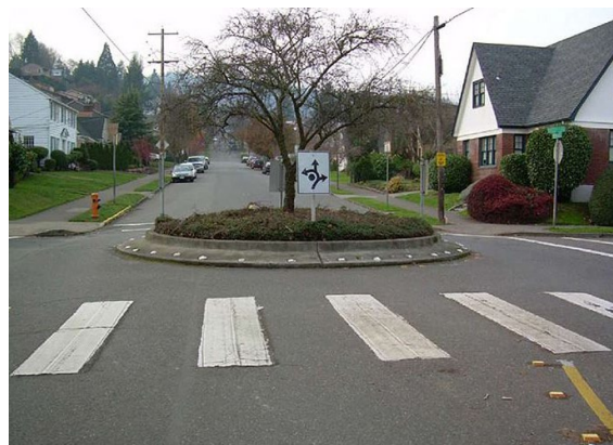
Traffic circle with landscaping. Source: U.S. DOT FHWA, Speed Management, Traffic Calming.
