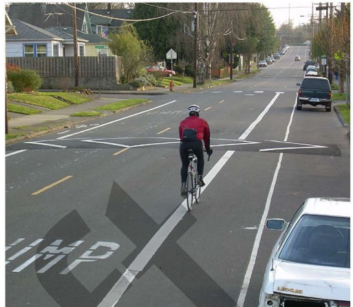
Speed hump on a street with bike lanes and on-street parking. Source: U.S. DOT FHWA, Speed Management, Traffic Calming.
