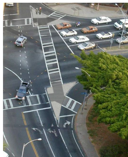
Example of a well-designed right turn slip lane. Source: Pedsafe, U.S. DOT FHWA.
