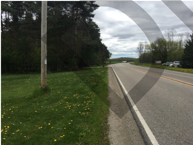
Looking east, the narrow right-of-way and no paved shoulder along Centennial Centre Boulevard between Forest Road and Oakview Court. Source: BC Planning Commission.
