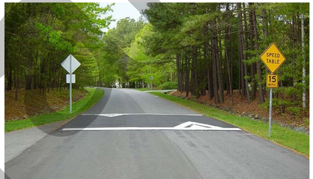
Speed table. Source: U.S. DOT FHWA, Speed Management, Traffic Calming.
